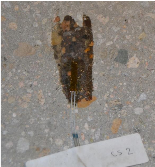
Figure 73 - Strain Gage Attached to Top of Slab (July 2014)
