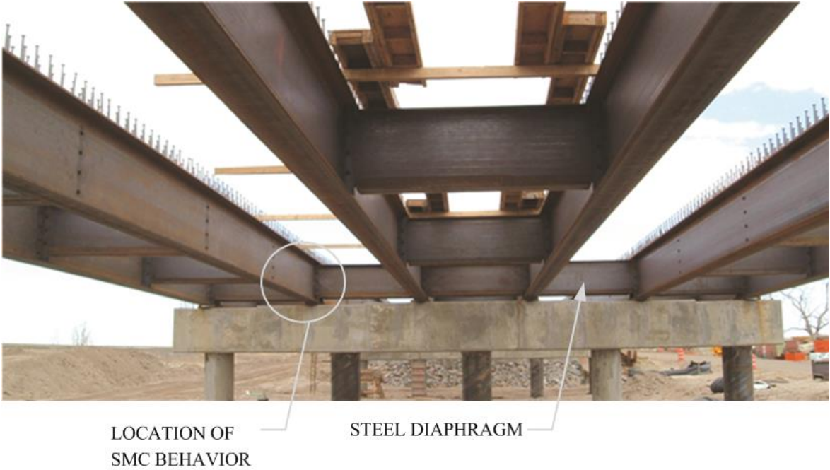
Figure 22 - SH 36 Over Box Elder Creek – Girder Details (reprinted courtesy of AISC)
