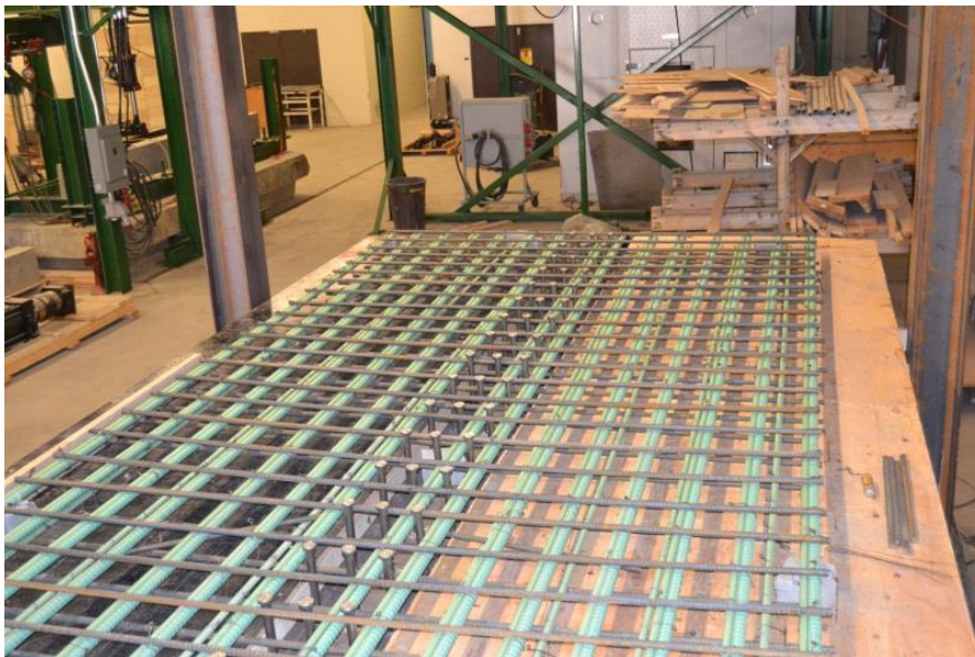
Figure 62 - Slab Reinforcing Placement (March 2014)
