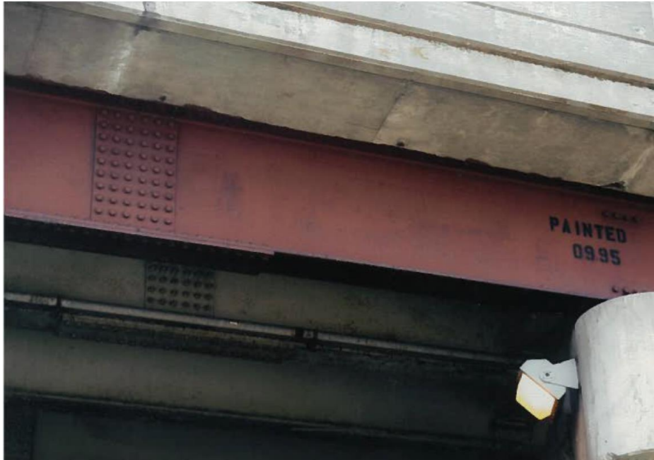
Figure 2 - Typical Continuous Girder Bridge Bolted Splice over Roadway
