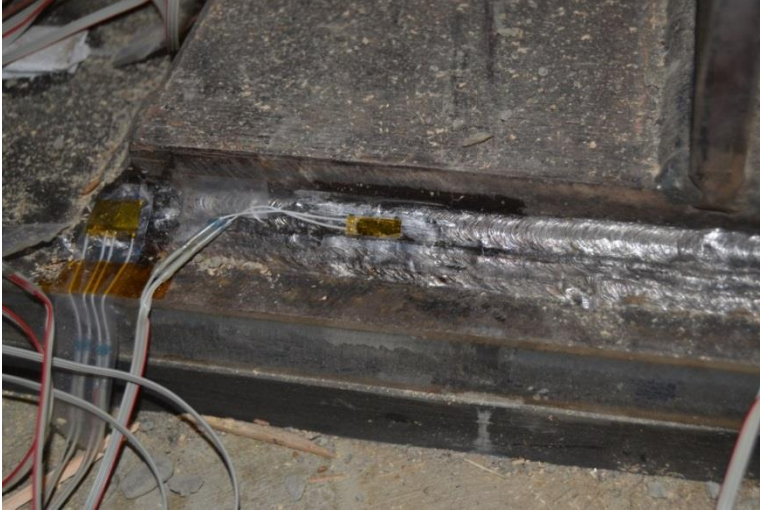
Figure 72 - Gage Placement at 5/8" Sole Plate Fillet Weld (July 2014)
