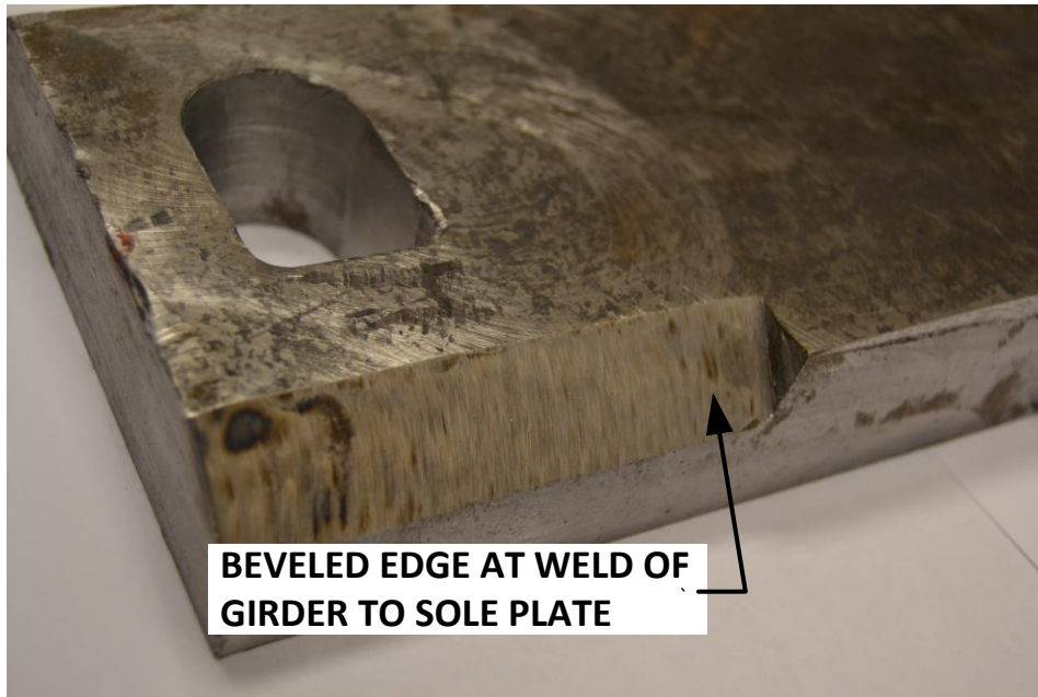
Figure 99 - Detail of Safety Device Showing Bevel at Weld
