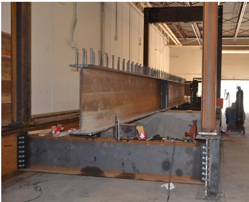
Figure 60 - Bridge Girders with Studs (March 2014)
