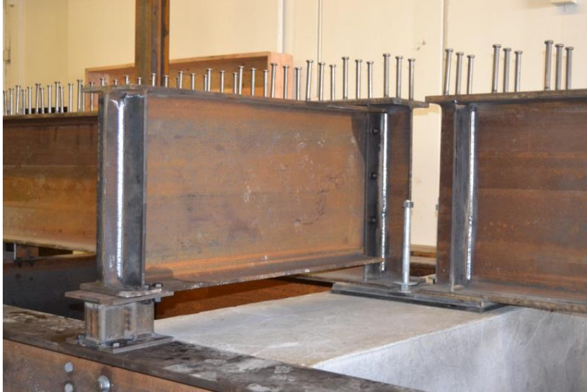
Figure 61 - Steel Diaphragm Beam (March 2014)
