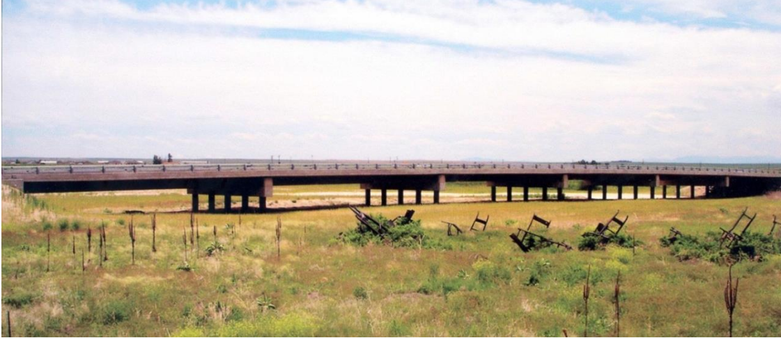
Figure 21 - SH 36 Over Box Elder Creek (reprinted courtesy of AISC)
