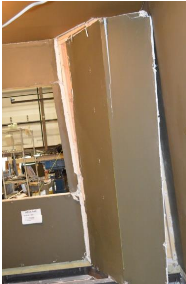
Figure 5-17: Damage State 4 and Damage State 5 Example
