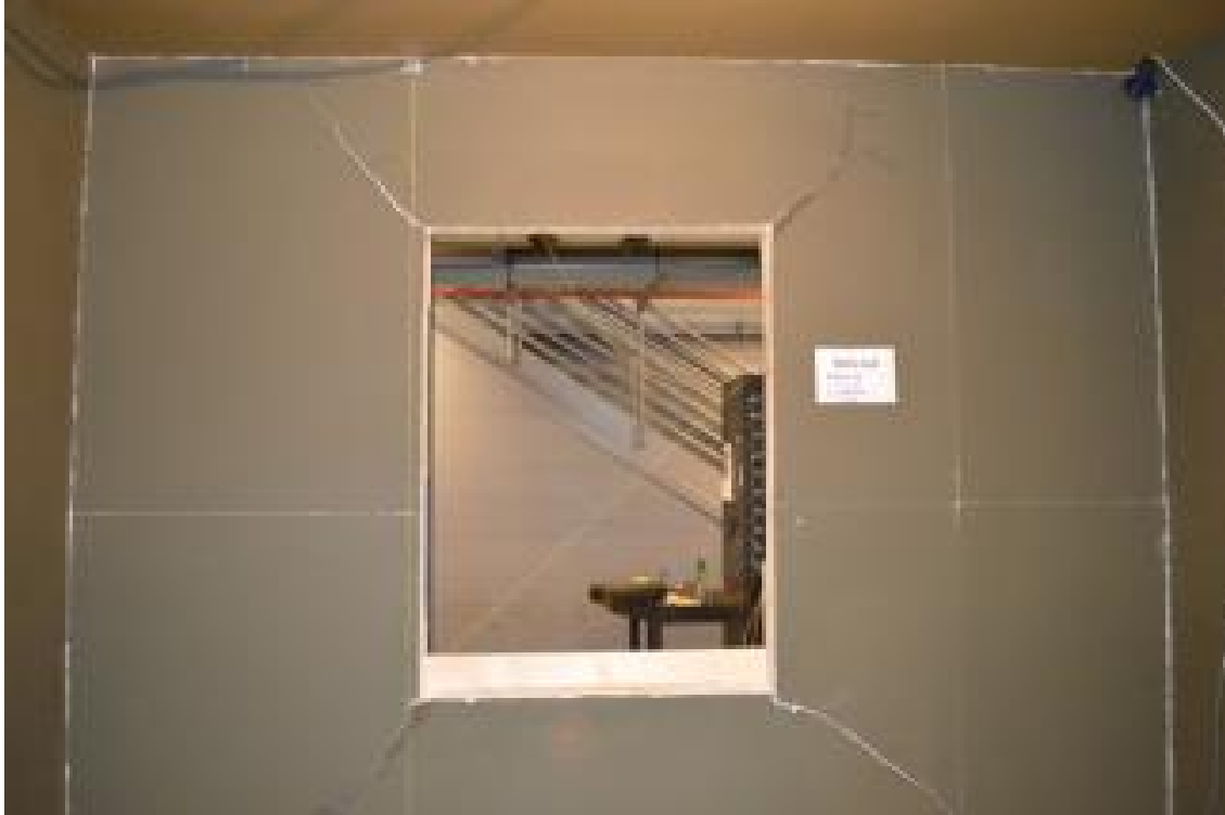
Figure 5-16: Damage State 3 Example
