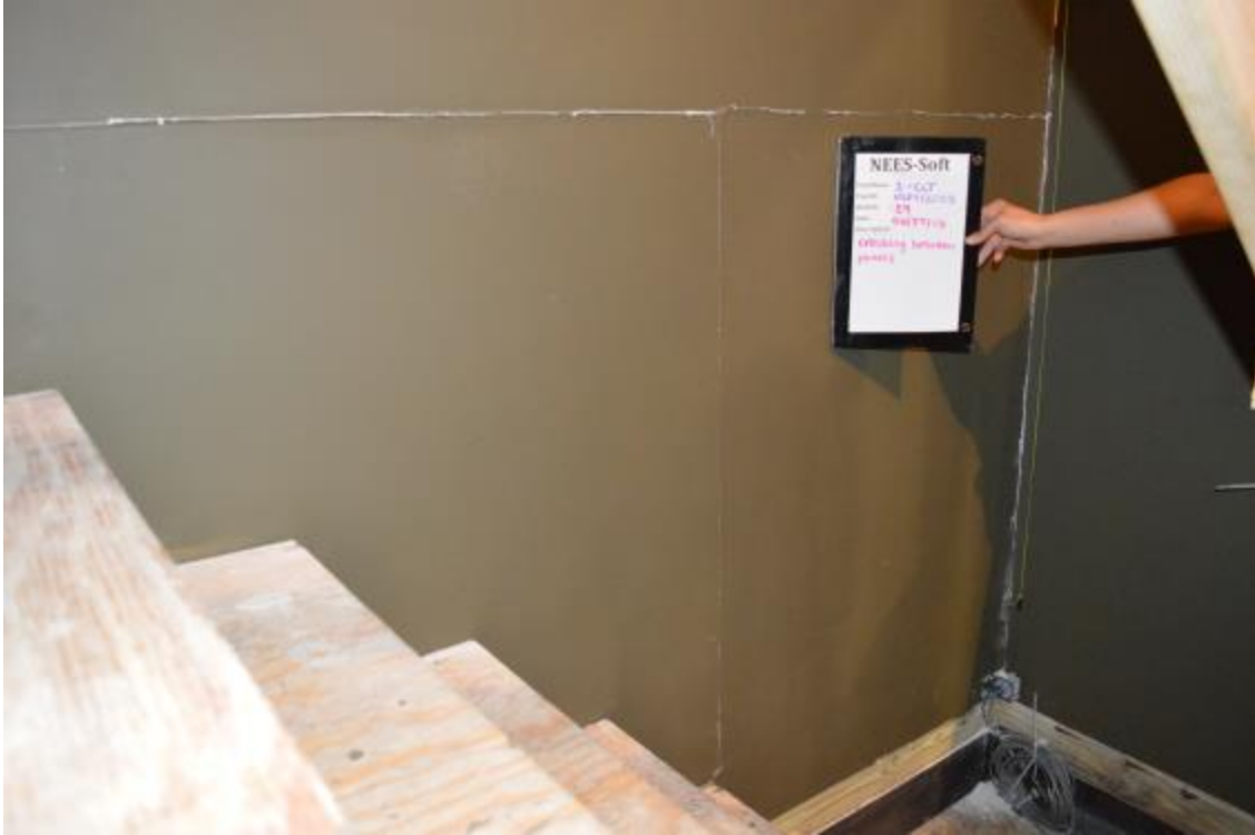
Figure 5-15: Damage State 2 Example
