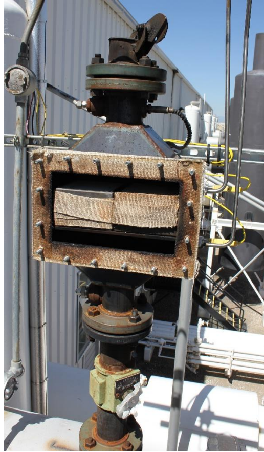
Figure 2.5: Initial Field Catalyst Slipstream Assembly
