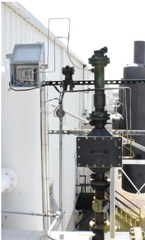
Figure 2.6: Field Catalyst Slipstream Assembly with Pitot Tube
