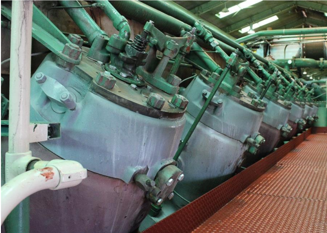
Figure 2.2: Field Cooper Bessemer GMVH-12 Engine
