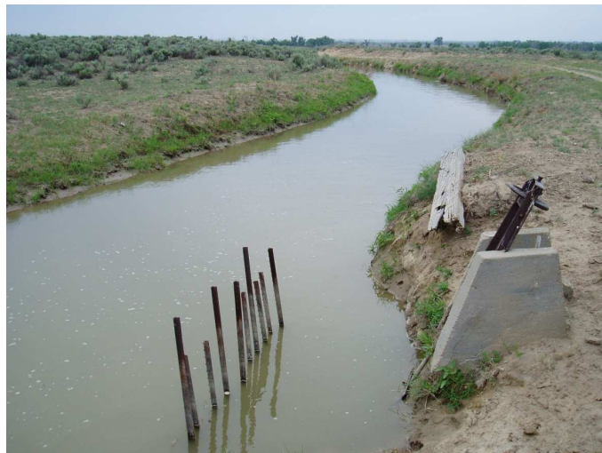
Figure 2-8 Photograph of a typical section of the Lamar Canal study reach (2006)
