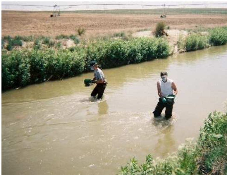
Figure 4-3 PAM application on the RFH Canal by walking the canal with handheld spreaders
