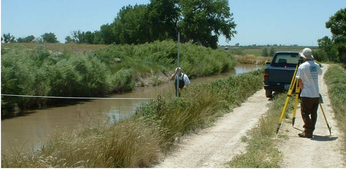
Figure 3-10 Cross-sectional survey on the Catlin Canal using a surveying level
