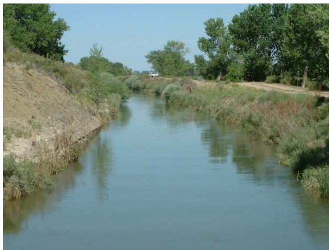
Figure 2-3 Photograph the RFH Canal between stations 201 and 202 (2006)
