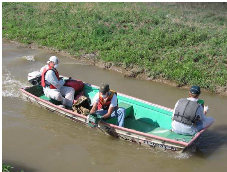
Figure 4-2 PAM application with a boat on the Lamar Canal using handheld spreaders
