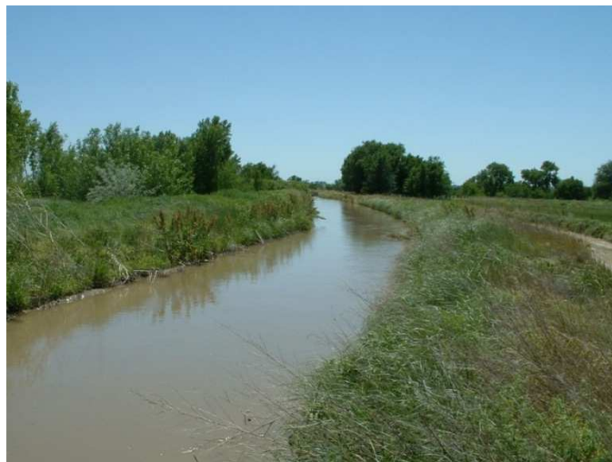
Figure 2-5 Photograph of a typical section of the Catlin Canal study reach (2006)
