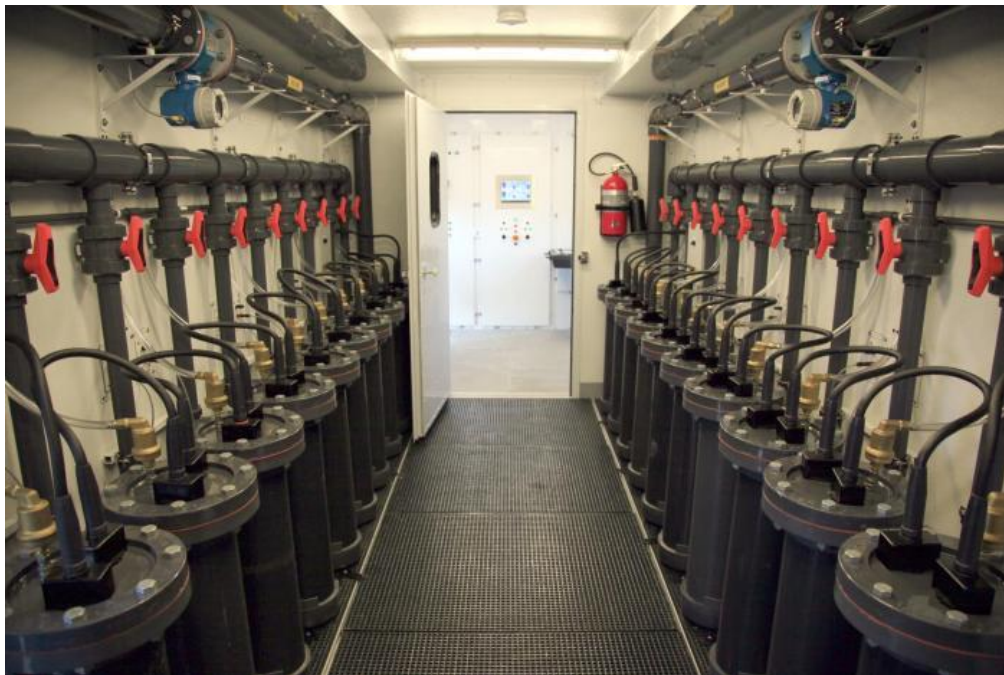
Figure 27. Inside view of the mobile EC trailer. Courtesy of Halliburton.
