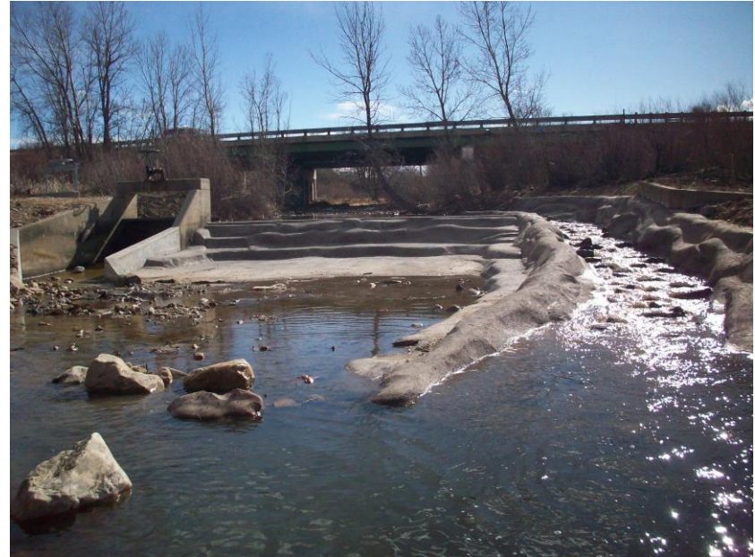
Figure 4-1. —The model rock ramp constructed at the Colorado State Engineering Research Center (left photo) and an example of a low-flow notch in a fishway in a small Colorado stream (right photo). The low-flow notch in the fishway is 21.3 m long and has a slope of 4.5%. The model rock ramp fishway was constructed in a 1.2-m wide flume, and average water depths were 0.11 m.
