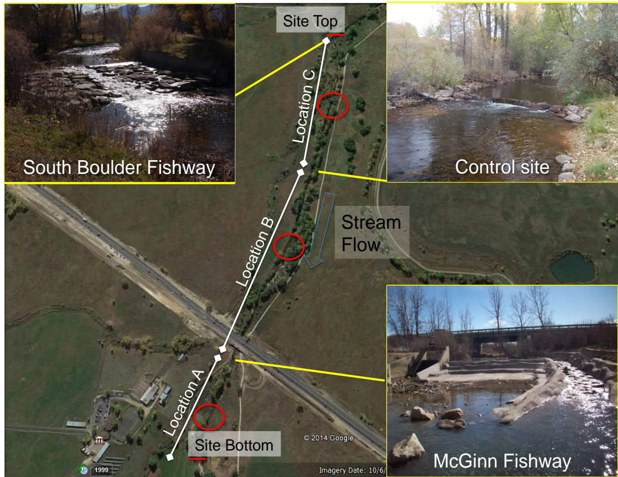
Figure 5-1. —The South Boulder Creek study segment. The two fishways are 0.9 km apart. McGinn Diversion (downstream) has a lower slope (4.5%) and a confined low-flow notch; South Boulder Ditch Diversion (upstream) has a higher slope (11.2%) and an unconfined low-flow notch. Locations A, B, and C refer to stream sections below the McGinn fishway, between the McGinn fishway and the control site, and between the control site and the South Boulder fishway, respectively. The circles indicate fish release locations after tagging.
