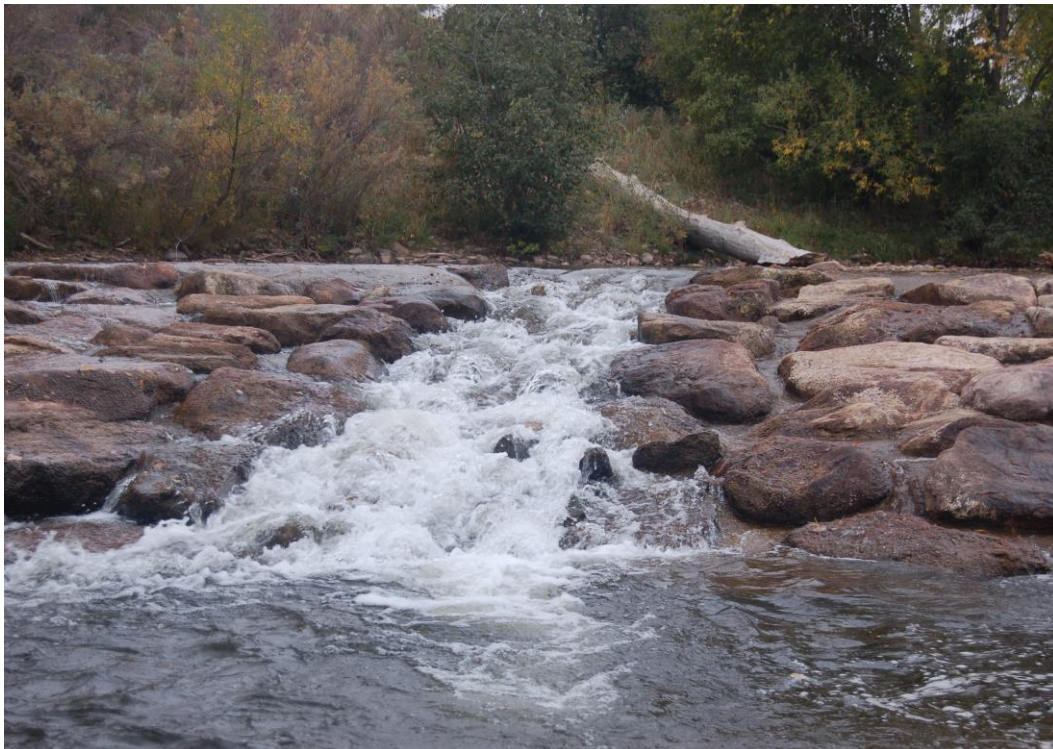
Figure 5-2. —The McGinn fishway (top) and South Boulder fishway (bottom). Although water overtops the entire McGinn structure at high flows, the low-flow notch shown in the photo (top right) is characterized by high velocities during high flows.
