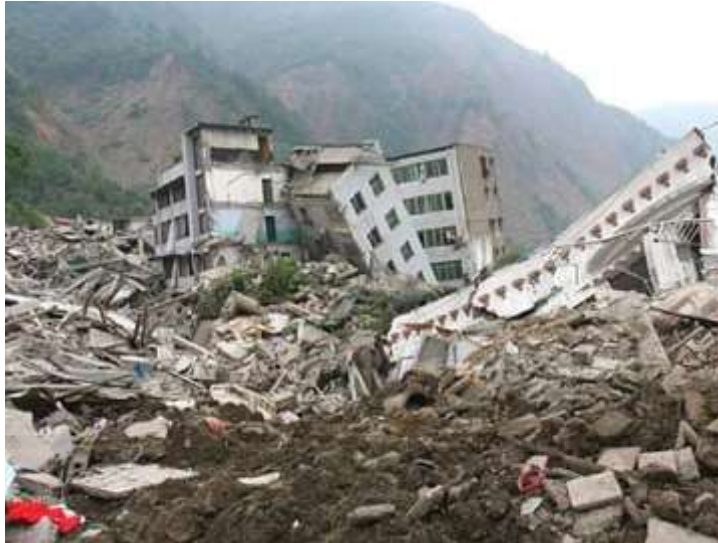
Figure 1.6 Building devastation from the 2008 Wenchuan earthquake in China; URL: ( http://www.iris.edu/gallery3/research/lrsp/SB5b )
