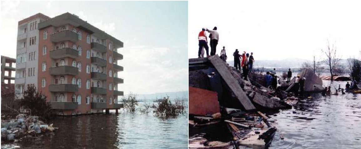
Figure 1.10 Multistory residential building in Gölcük, Turkey (a) The survived building after the mainshock (b) The same collapsed building in the M5.9 aftershock one month after the mainshock (photos are excerpted from USGS, 2000)
