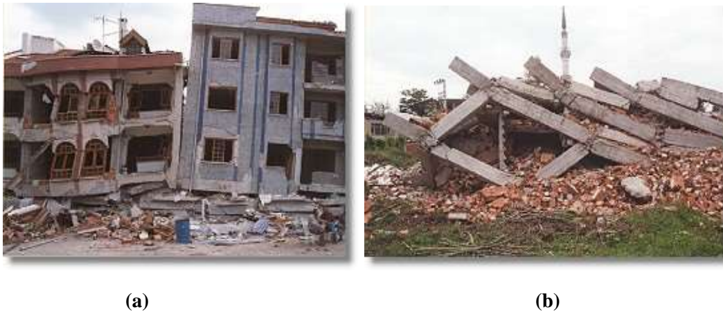
Figure 1.8 Building collapses during the Turkey Kocaeli earthquake (a) Collapse of the first story and damage due to pounding between adjacent buildings (b) Total collapse of a building because of inadequate design at the beam-column joints; URL: ( http://whatiscivilengineering.csce.ca/structural_earthquakes2.htm )
