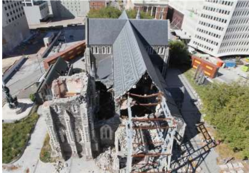
Figure 1.5 Damaged Christchurch Cathedral after the earthquake; URL: ( http://www.odt.co.nz/news/dunedin/209566/city-councillor-explains-significance-peoples-place )
