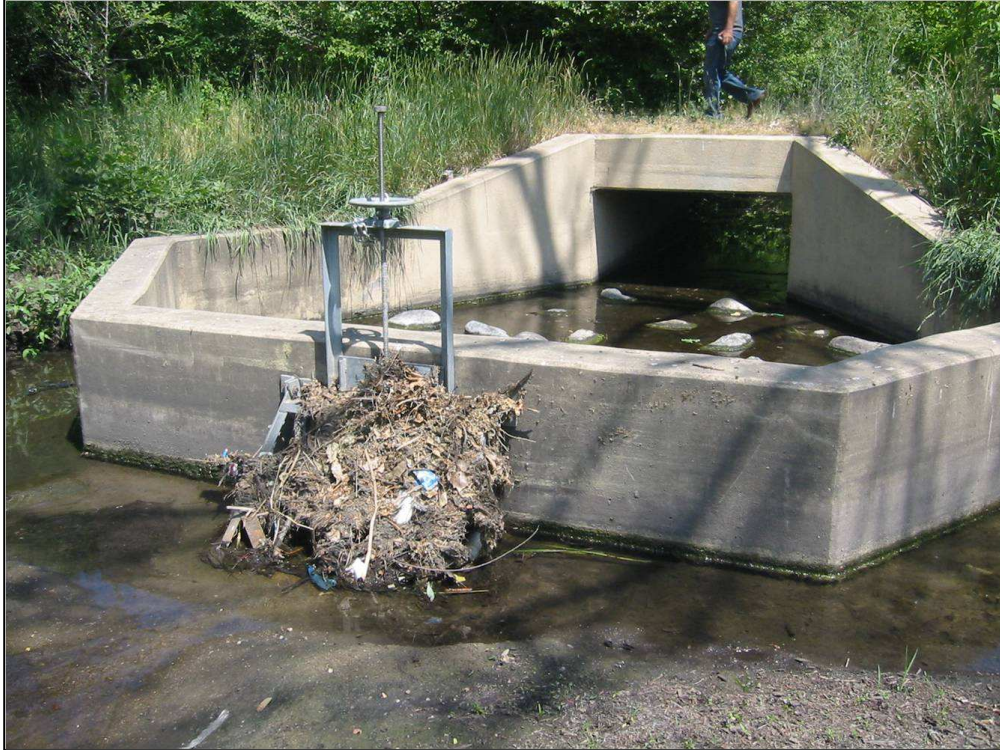
Figure 3.4. The Howes Street Basin wetland water quality control structure located at the outlet of Cell 1
