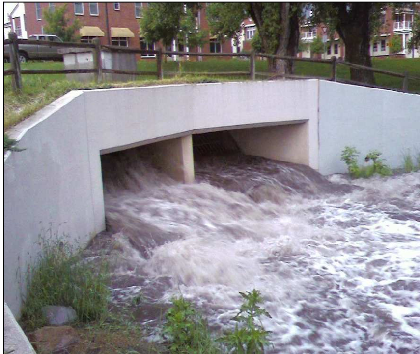
Figure 3.3. The Howes Street Basin main outlet to the wetland, a 20ft by 20ft double box culvert
