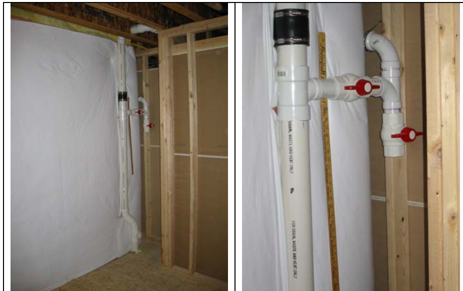
Figure B-1: Residential graywater system connection point
