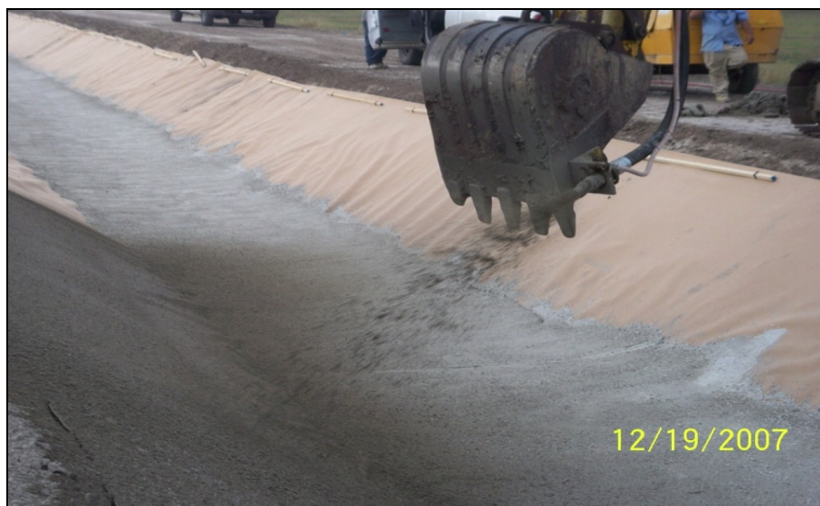
Figure 15. Shotcrete being sprayed onto the fibrous polyester liner
