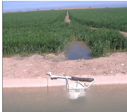
Figure 8. Linear actuator in operation on a turnout gate at Imperial Irrigation District automated surface irrigation demonstration site
