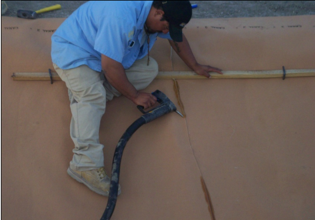
Figure 10. Glues being applied to the joints of a polyester liner.
