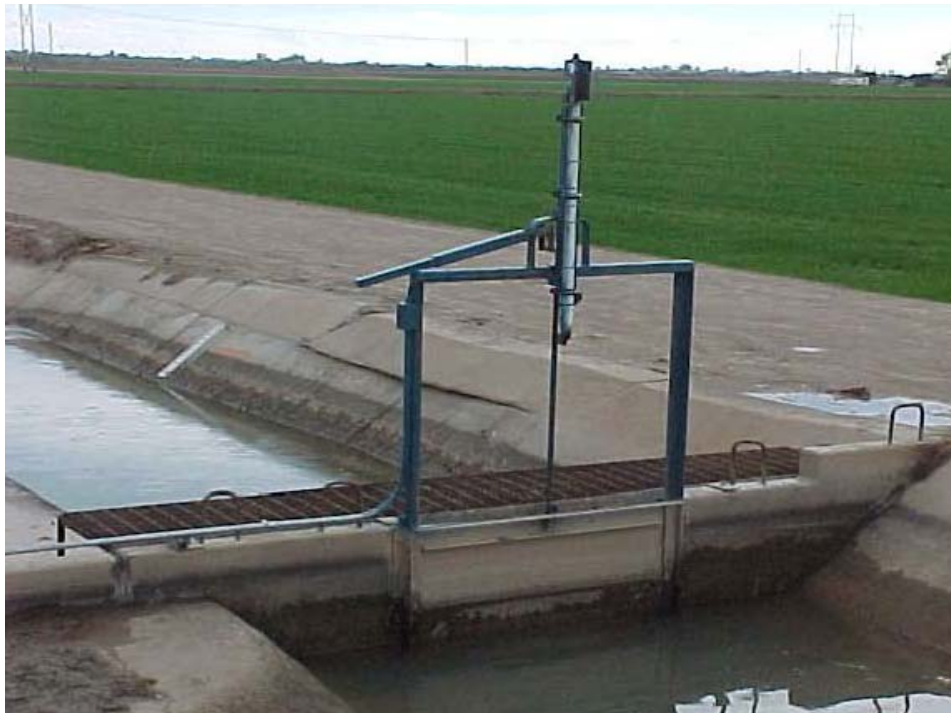
Figure 2. A vertical slide gate with a linear actuator installed
