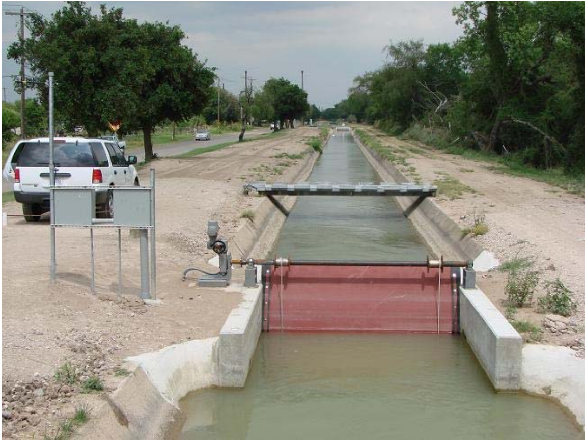
Figure 3. New radial gate and structure.
