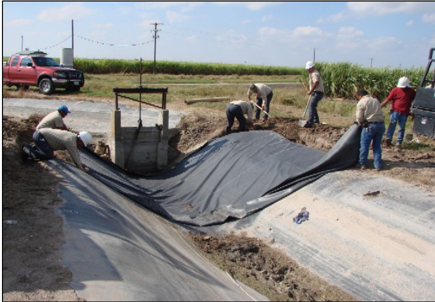
Figure 16. A district maintenance crew repairing a damage section of lining
