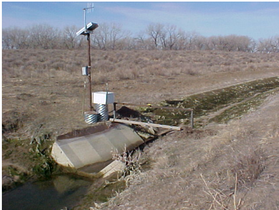
Figure 1. 2005 Photo of the SPDC G2 Flume
