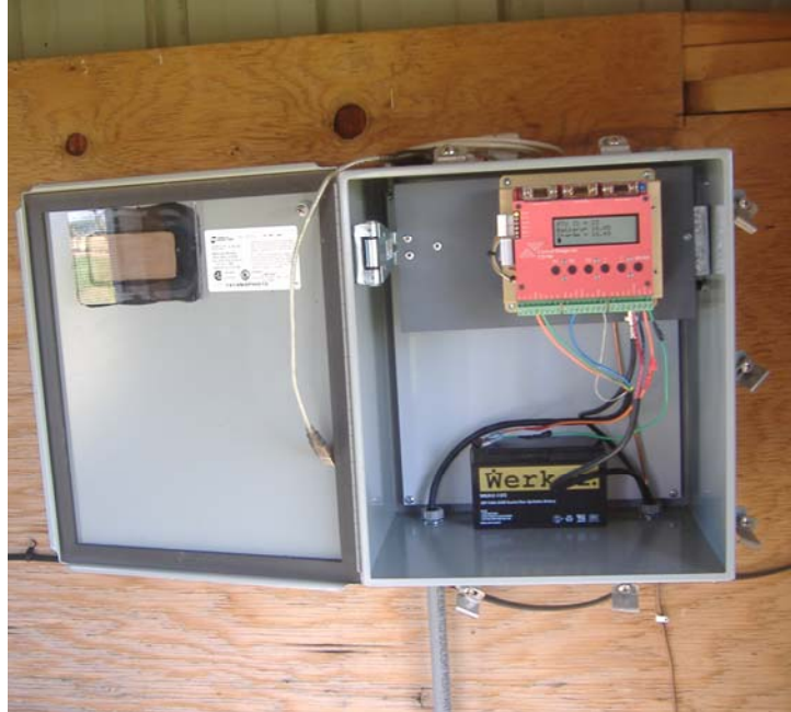
Figure 6. A CDI Radio/Control Unit Installed in the Pump House Shown in Figure 5
