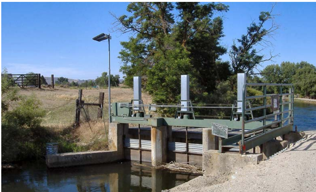
Figure 2. Farmers Cooperative Automated "Squeeze Gate" Structure
