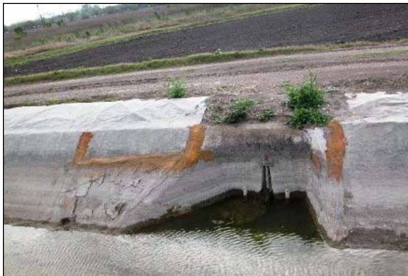
Figure 17. Repair of the liner joints around a structure with glue
