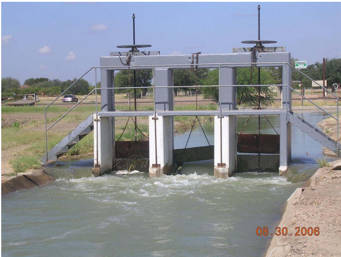
Figure 2. Pre-existing head slide vertical gate structure of the Bryan canal.
