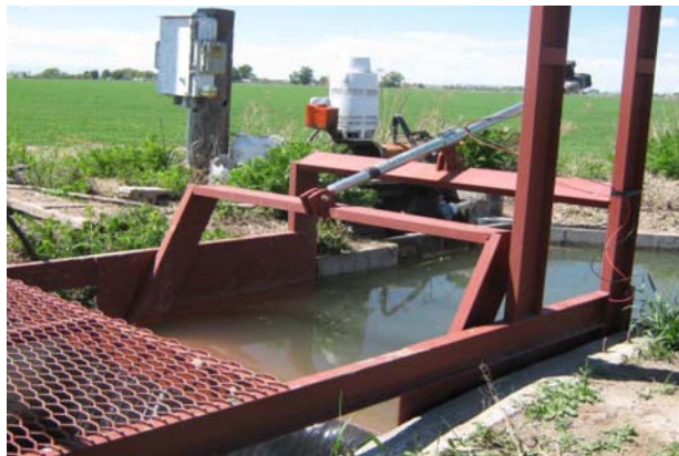
Figure 11. Self-constructed overshot gate in eastern Idaho.
