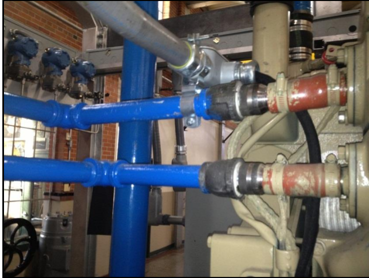
Figure 10. Intercooler Coolant Connections.
