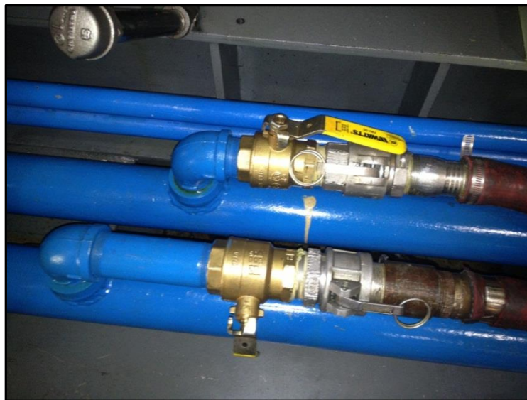
Figure 8. Catalyst Testing Unit Coolant Connections.
