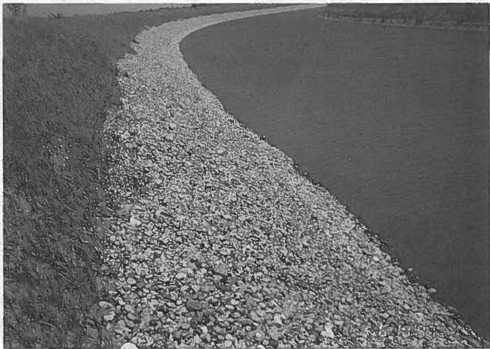
Fig. 12. The beach belting placement is complete.
