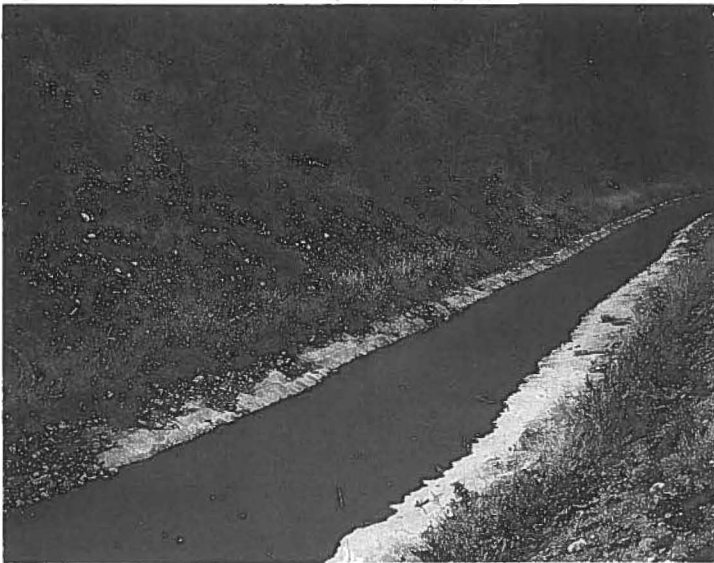
Fig. 2 Plastic lining of a rock/earth canal
