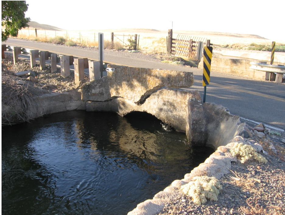
Figure 2. OID North Main Canal Conduit Crossing at Sonora Road
