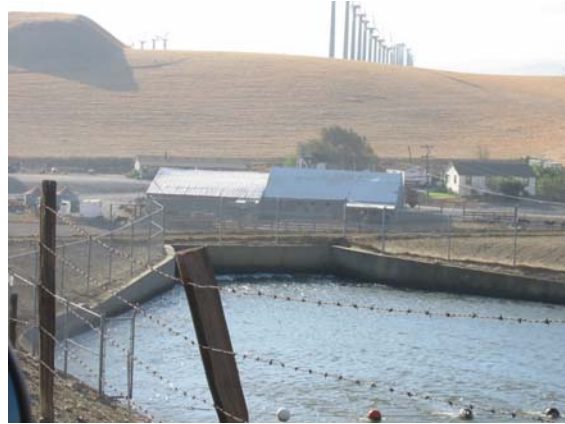
Figure 4. Inverted Siphon Entrance
