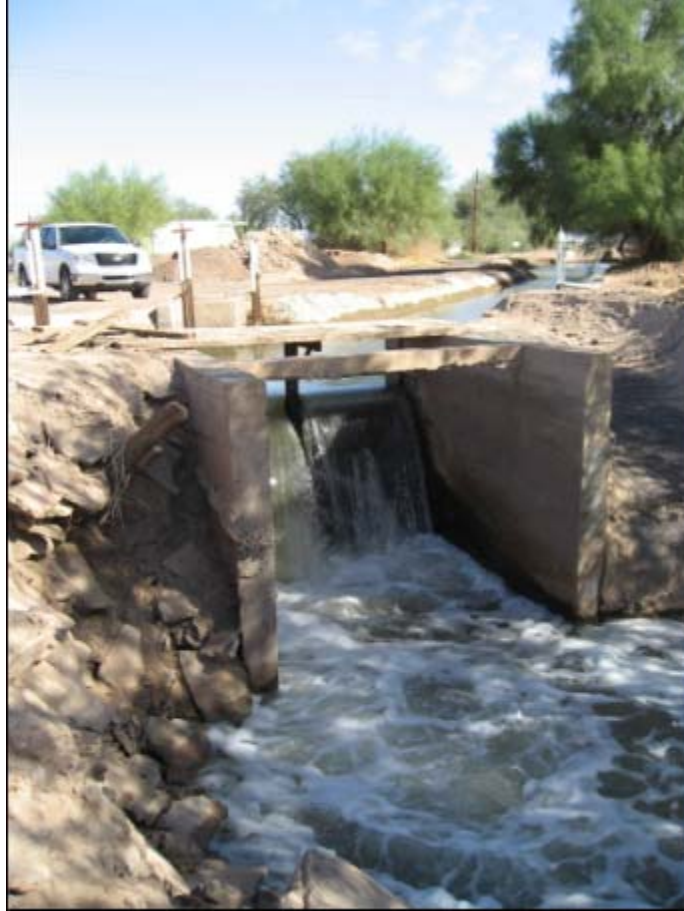
Figure 1. South Extension canal drop
