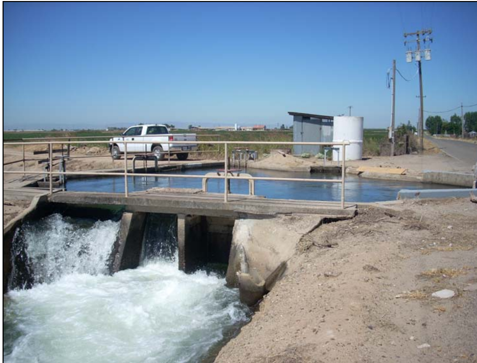
Figure 2. Downstream View of Typical OID Diversion Structure
