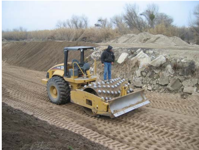
Figure 4. Ride-on vibratory compactor for bottom of canals.
