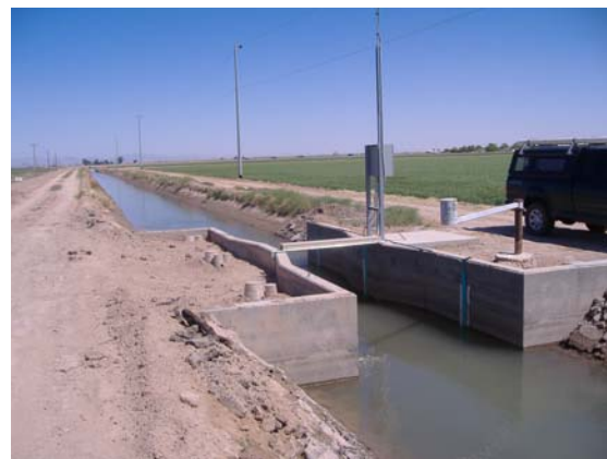
Figure 7. YCWUA Cumming Flume
