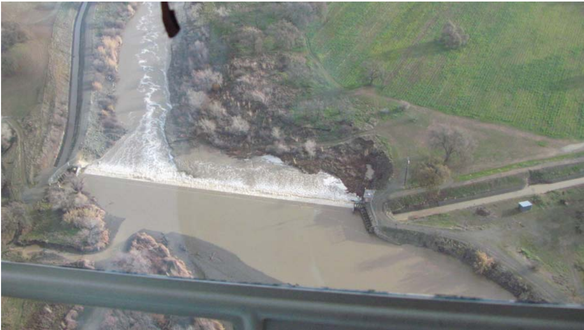
Figure 2. Aerial Photo of Capay Diversion Dam
