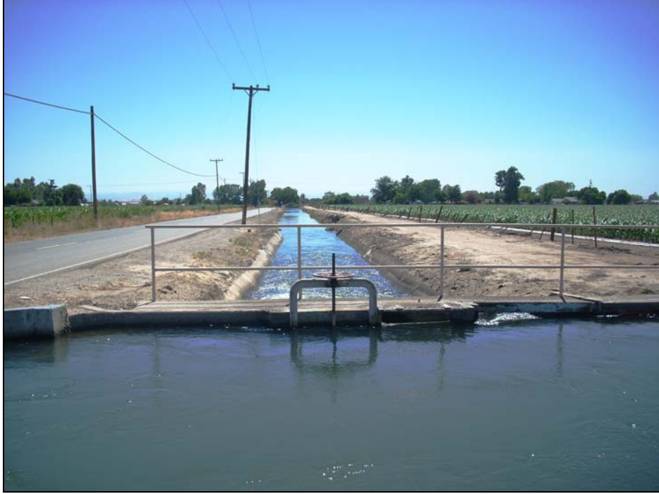
Figure 1. Upstream View of Typical OID Diversion Structure
