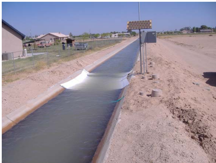
Figure 4. Unit B District Flume
