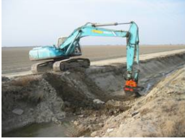
Figure 7. Compacting the sides and bottom of Lateral H at James ID
