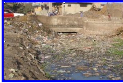
Figure 3. Canal Infestation with Solid Wastes
