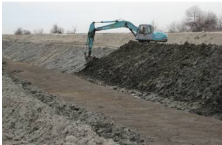
Figure 3. James ID Main Canal during side compaction
