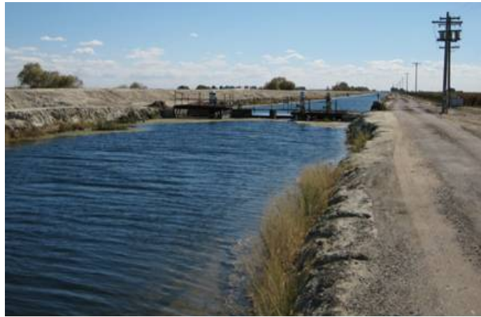
Figure 2. James ID Main Canal during pre-compaction seepage test
