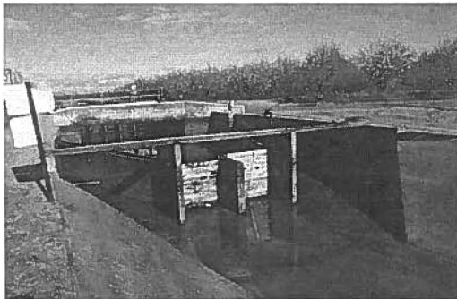
Figure 4 - Long Crested Weir
