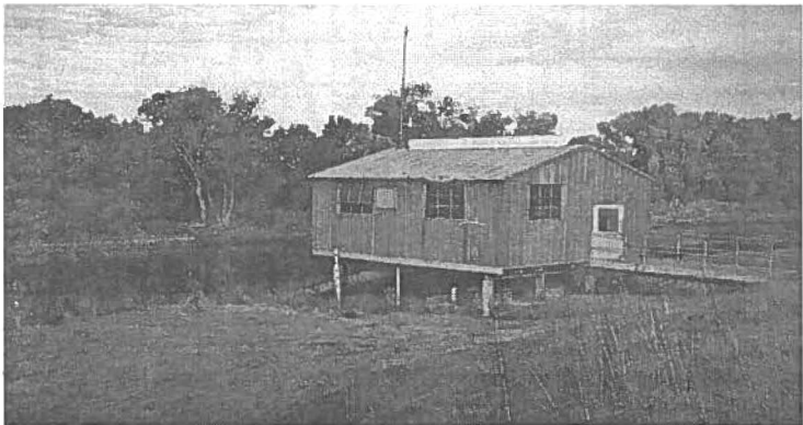
Figure 2: Portuguese Bend Pumping Plant on the Sacramento River
