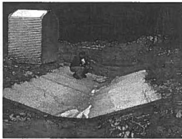
Figure 6. Triangular-Throated Flume in Florida.
