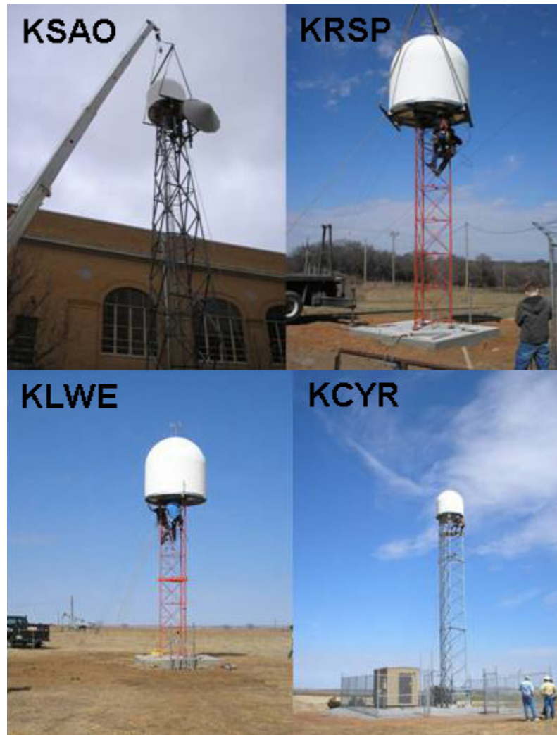
Figure 5. The four polarimetric radars forming the CASA radar network.
