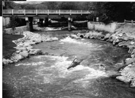
Figure 20. Stream changes in an urban corridor along Boulder Creek.
