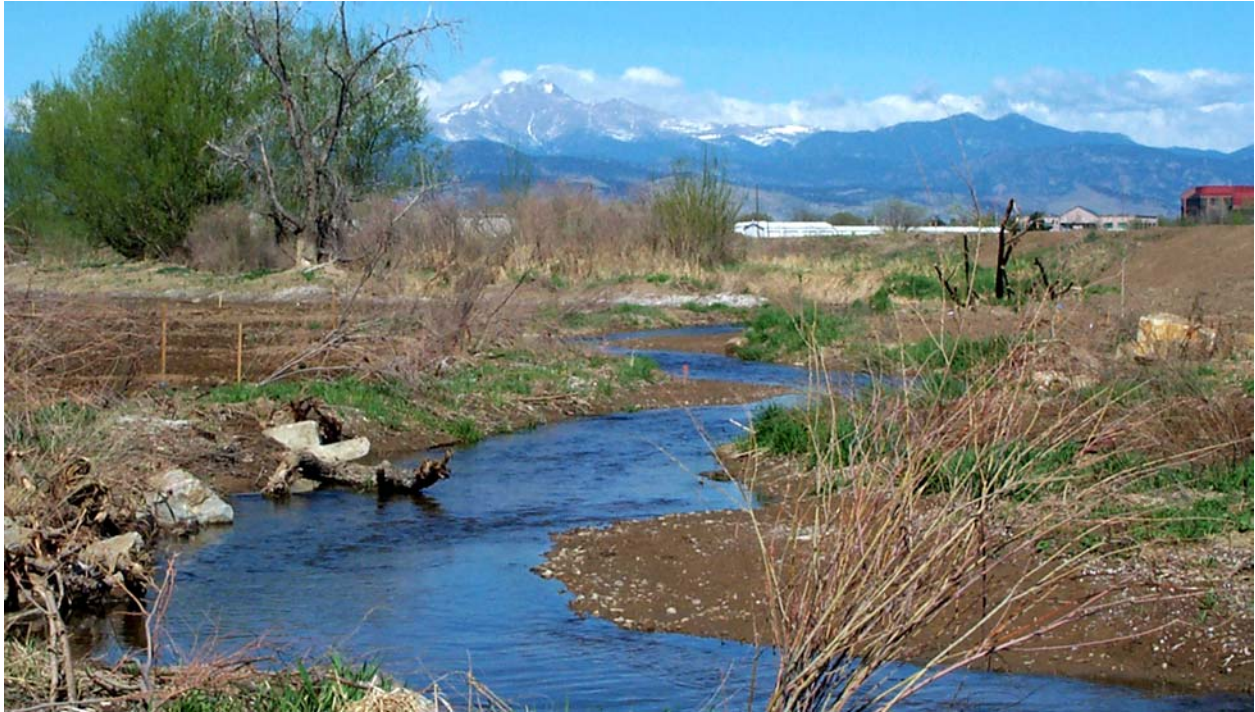
New Lefthand Creek Channel, 2002, view to west. Note streambanks stabilized with willow plantings, root wads, and boulders.
