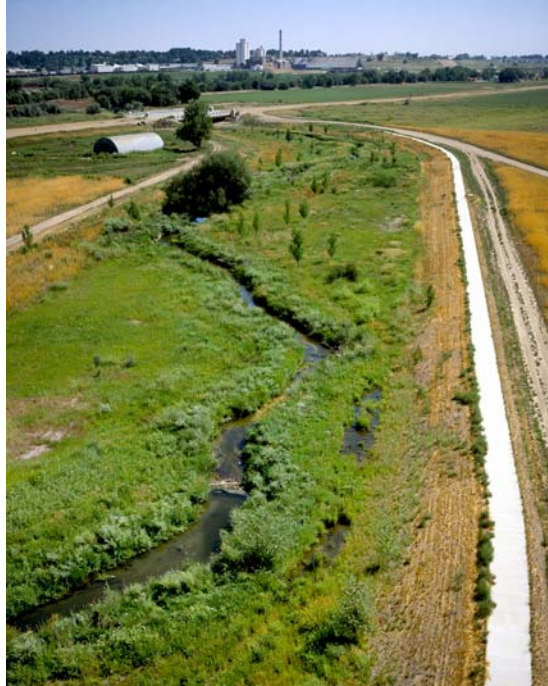
Lefthand Creek, summer 2003, oblique aerial view to east. Note stream meanders, developing wetlands and landscape plantings. Ken Pratt Boulevard Bridge in background, trail at right.
