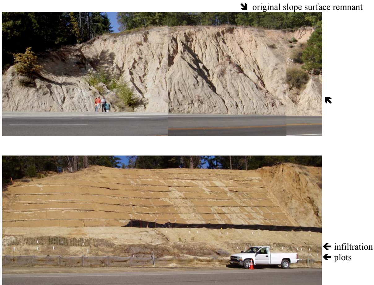
Figure 1. (top) Field study site before treatment. Note gullies resulting from sealed slope surface and overland flow. Bare area behind the center slope is an old logging landing which percolates water down into the decomposed granite batholith, where it runs laterally and pipes out at about two-thirds the way up the slope. Remnant slope surface showing original 40° grade is located at right of slope under arrow. (bottom) Same slope following treatment. Finished slope was covered with coir blanket (700 g/m 2 ), which was keyed across the top of each 1.5 m lift. Rainfall simulation plots are located at the lower part of the slope left of the double arrows (left of double arrows).
