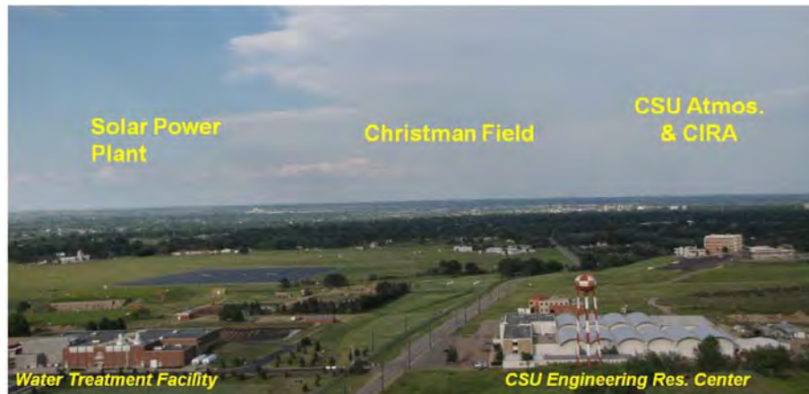
Figure 1. The Colorado State University Foothills Campus will be used as a validation site. A 15 acre, ~2 MW solar power plant was built by Xcel Energy in 2009 and operated by Renewable Ventures.
