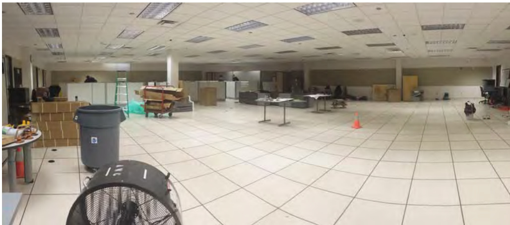
Figure 3. Complete tear down of OPS floor.
