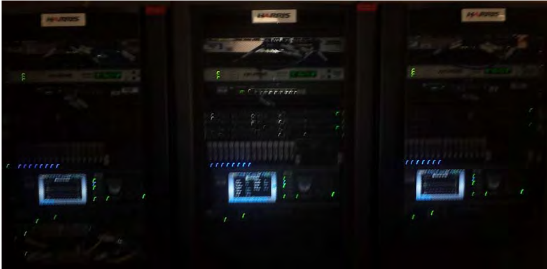
Figure 7. Satellite Antenna Rack controllers.
