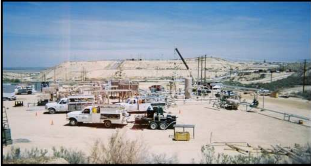
Figure 12: A photo of a rapid systems upgrade illustrating a coordinated upgrade
