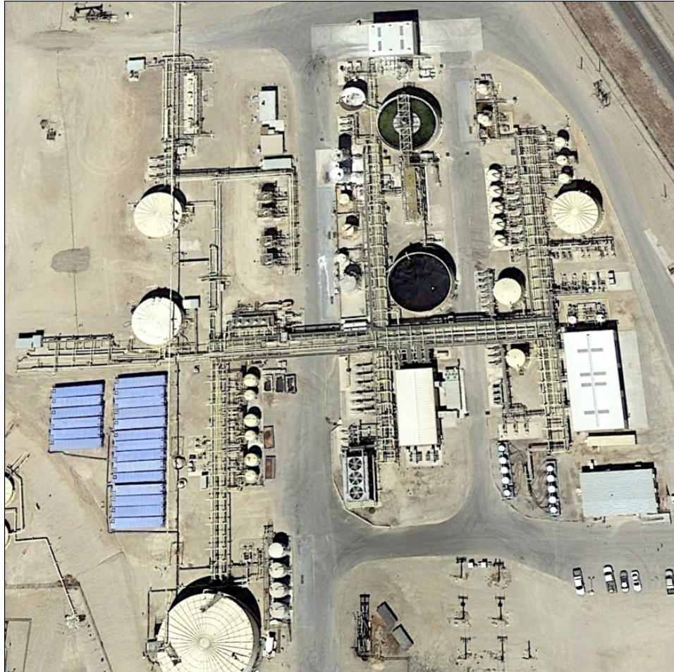
Figure 2: A typical heavy industry site illustrating a broad mix of process components
