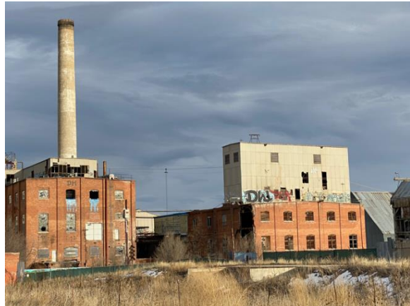
Image 2: View of the factory looking eastward.
