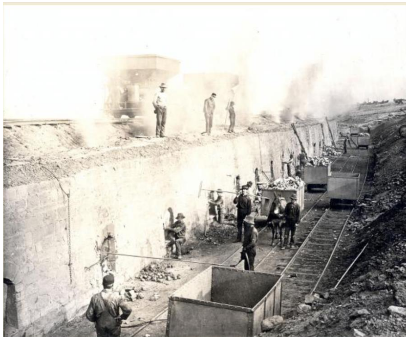
Figure 22: Beehive coke ovens in the Connellsville coke district, circa 1890, Courtesy of the Pennsylvania State Archives
