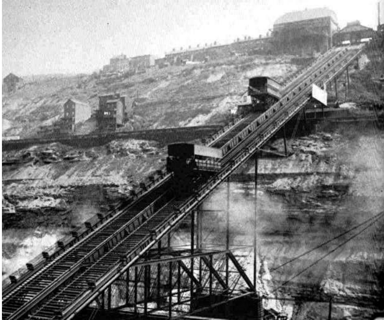
Figure 25: The Penn Incline, used to transport tons of coal from the extraction site on Mount Washington to rail cars and river barges. There are no trees and significant portions of the hill have been blasted away for coal as well as for the incline. A few houses of workers exist nearby. Library of Congress
