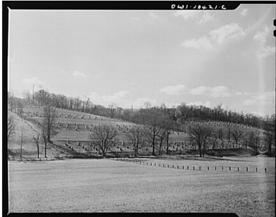
Figure 18: Pittsburgh, Pennsylvania (vicinity). Montour no. 4 mine of the Pittsburgh Coal Company. Above the coal seam, dairy and farmlands lay undisturbed. Only occasionally there will be "sinks" and large "potholes" caused by the collapsing of "mined out" areas of the seam. Image: Library of Congress
