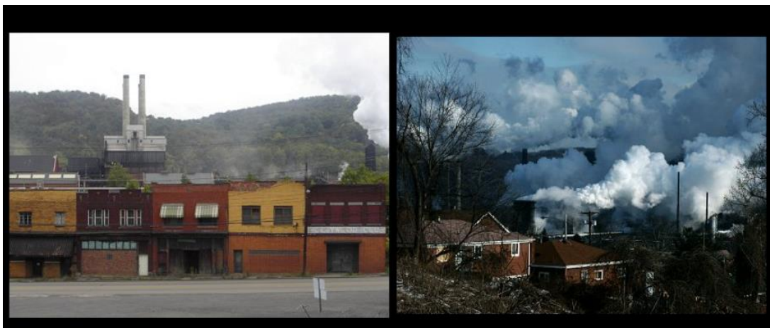
Figure 39: Mainstreet in Clairton, with works sitting abandoned. Figure 40: Clairton Coke Works, still in production today.
