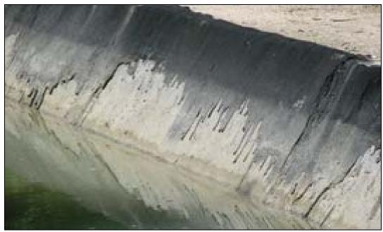
Figure 9. Residue left from a deteriorated polyurethane liner
