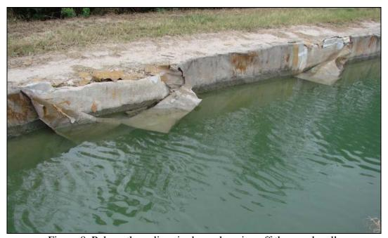
Figure 8. Polyurethane liner is shown hanging off the canal wall.
