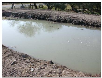
Figure 12. Water level higher than the canal liner installed
