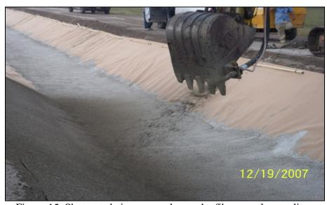
Figure 15. Shotcrete being sprayed onto the fibrous polyester liner
