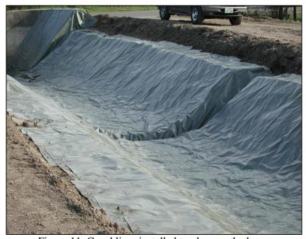
Figure 11. Canal liner installed too low on the levee
