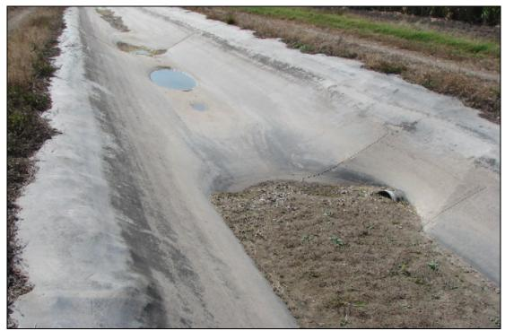
Figure 3. Aquatic vegetation and sedimentation clogging a farm outlet pipe
