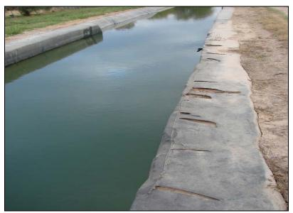
Figure 6. Cuts/tears in a rubber liner
