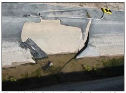
Figure 7. A rubber liner damaged possibly due to vandalism
