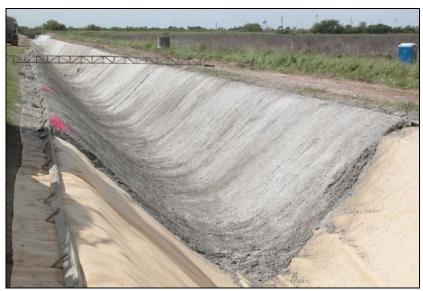
Figure 2. Polyester canal liner with a 3-inch protective barrier
