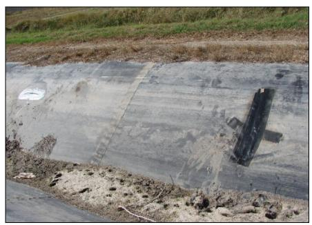
Figure 18. Sedimentation at the bottom of a lined canal
