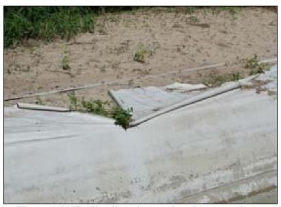
Figure 5. PVC Alloy liner damaged on the exposed area
