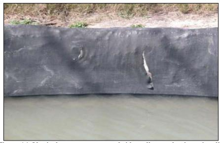
Figure 14. Vertical cut or tear on canal side wall caused unintentionally
