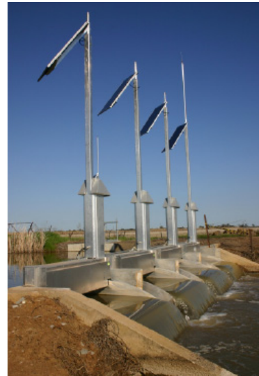
Figure 3. Repeater Tower: CICL SCADA Radio Network (left) and Canal Regulating Structure Equipped with Automatic Gates (right)
