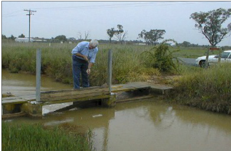
Figure 6. Manipulating Stop Logs in a Canal Regulator – Goulburn-Murray Irrigation District
