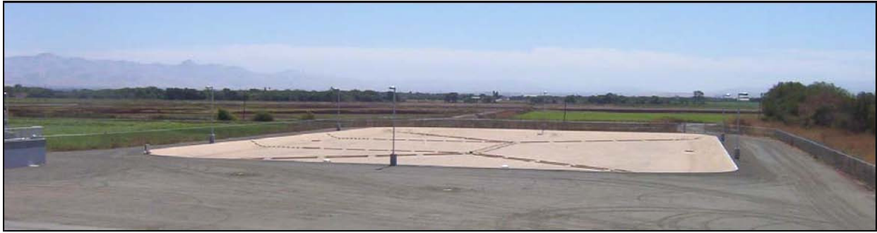
Figure 4. Photograph of Final Constructed Reservoir
