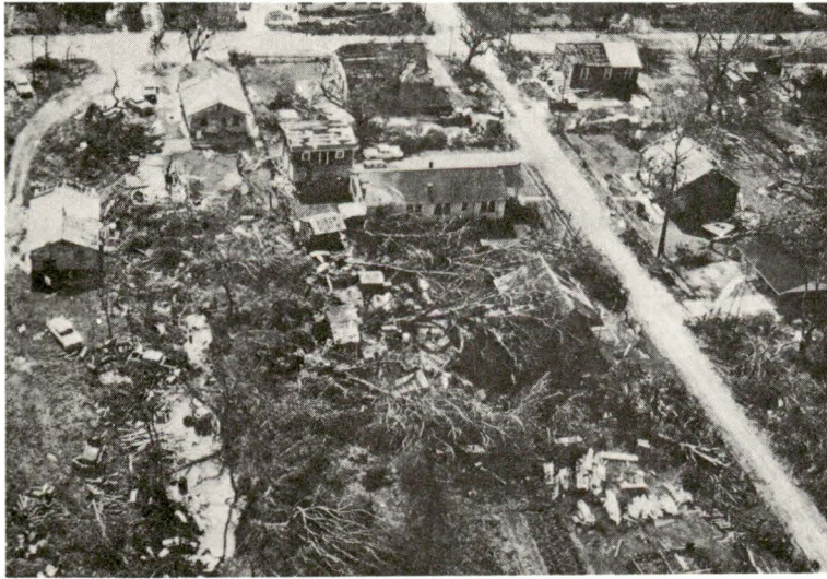
(a) Residential area in Bay St. Louis, Mississippi (Ref. 9)
