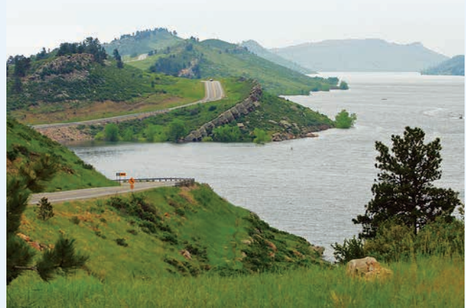
Horsetooth Reservoir. Photo by Fort Collins Utilities.
