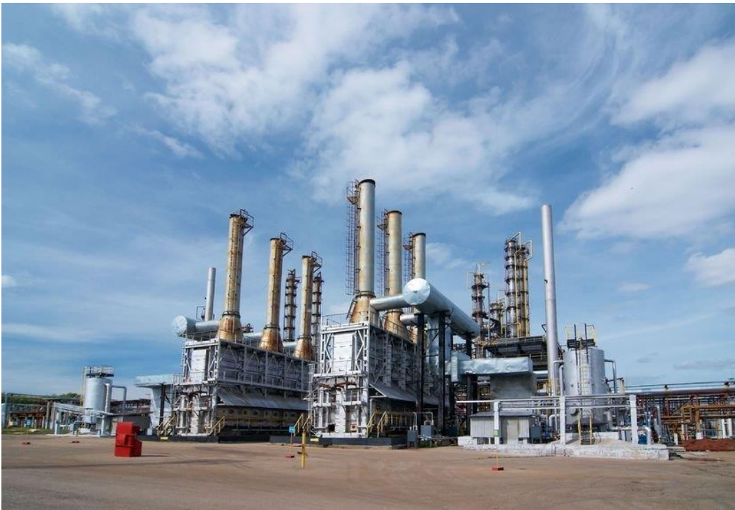
Figure 2-2: Natural Gas Processing Plant (source: https://www.bicmagazine.com )
