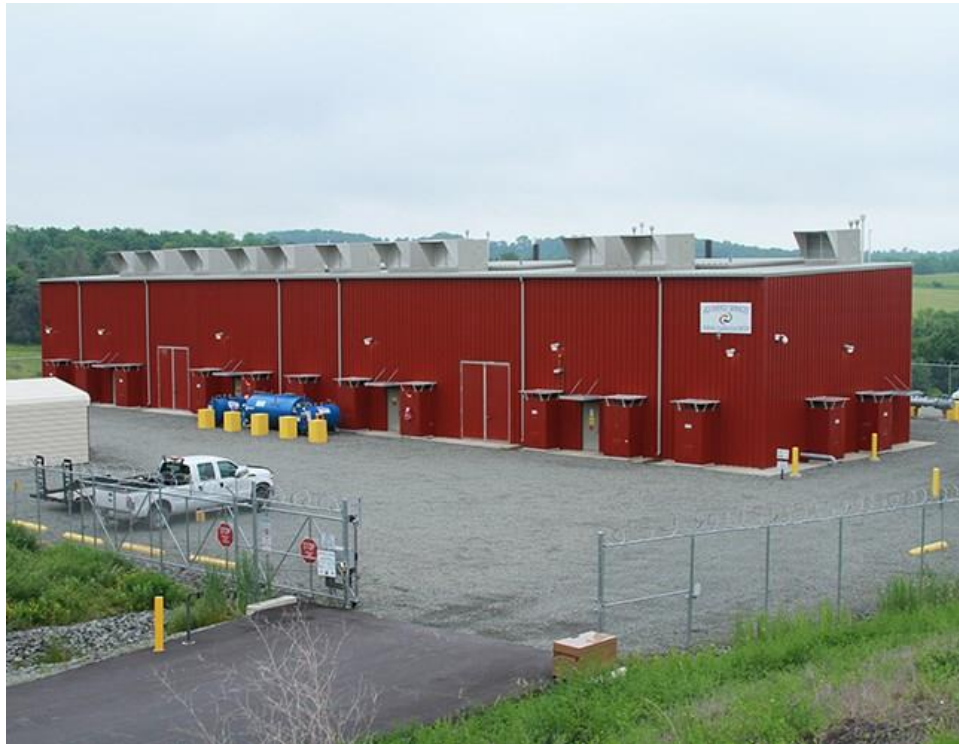
Figure 2-3: Exterior View of a Natural Gas Compressor Station (source: https://www.entecheng.com )
