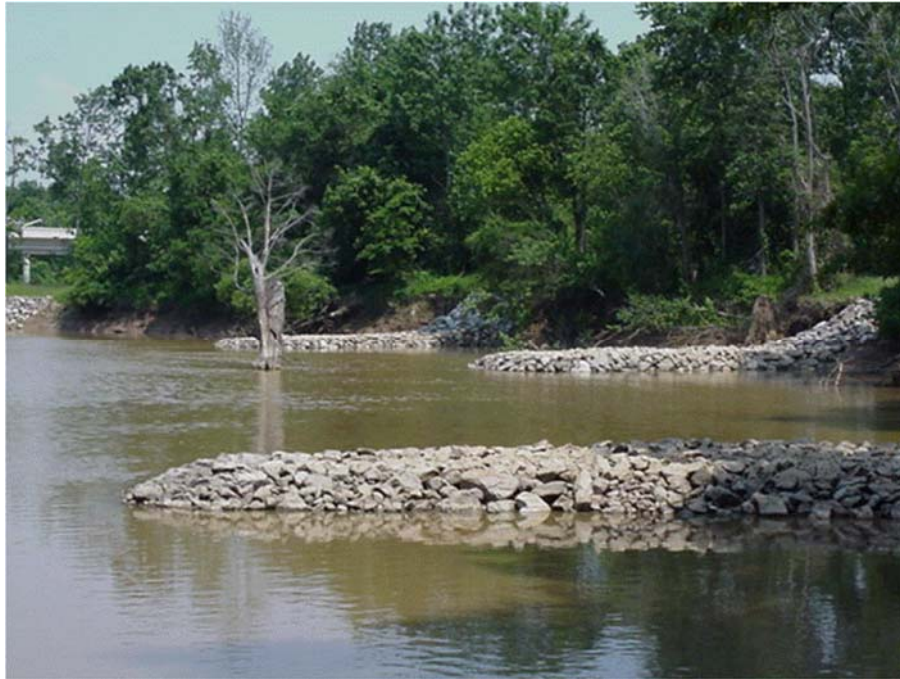
Figure 2: Bendway weirs installed in the field (Heintz 2002)
