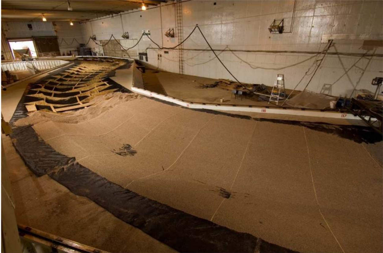
Figure 9: Construction of the simulated native bathymetry used in the hydraulic model (Scurlock 2014)
