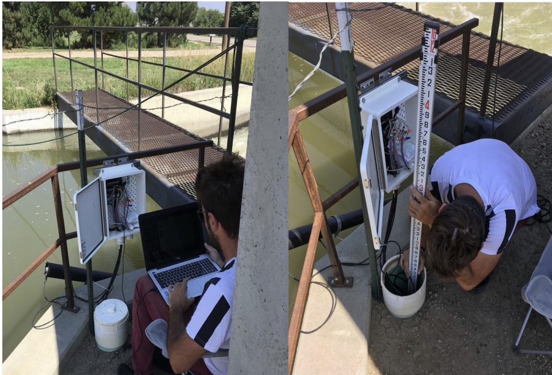
Figure 12. Water level measurements in the stilling well with a data acquisition system (left) and using a staff gauge at the stilling well at upstream of Gate B (right).
