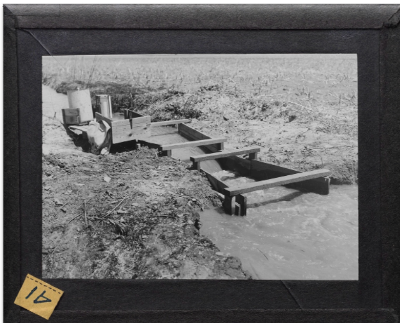
Flume developed by Ralph Parshall. From the Ralph L. Parshall Collection. Courtesy of the Water Resources Archive, Colorado State University.
