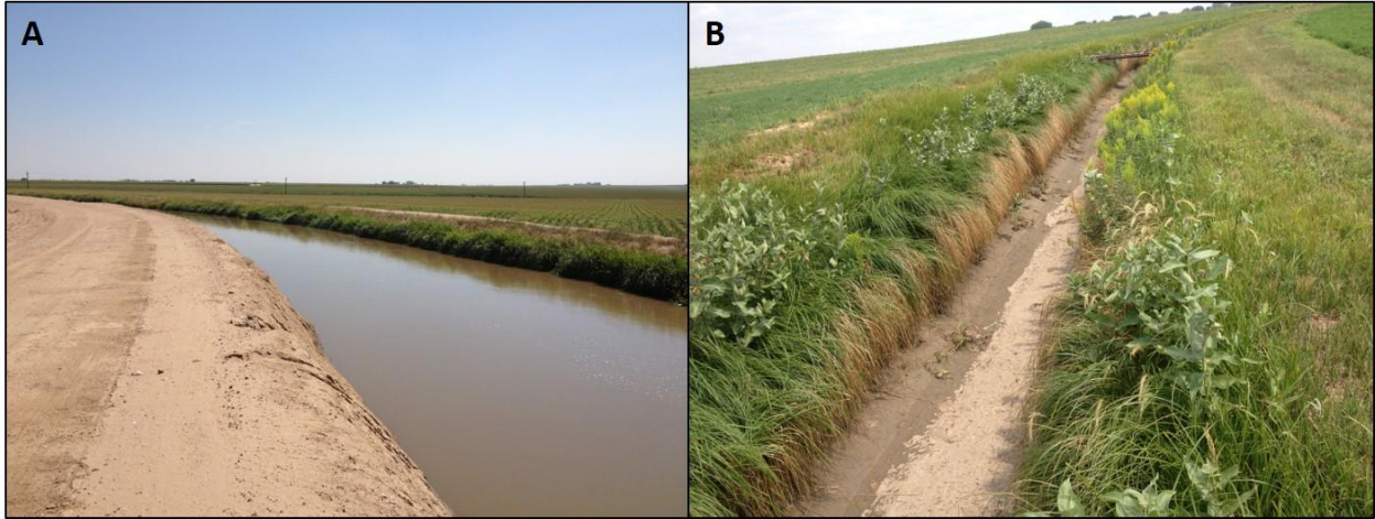
Figure 4.1: An example of a main stem canal (A) with significant vegetation management for road access and water conveyance, and (B) a small lateral ditch in Weld County, Colorado.
