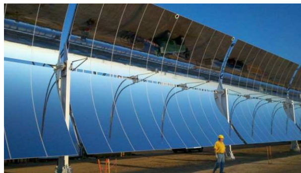
Fig. 8. Image of a parabolic trough collector (PTC) array with large aperture troughs. (Courtesy of Gossamer Innovations, gossamersf.com)
