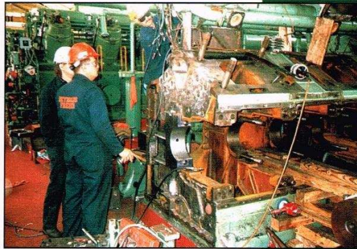
Above: Completed on-site repairs.
