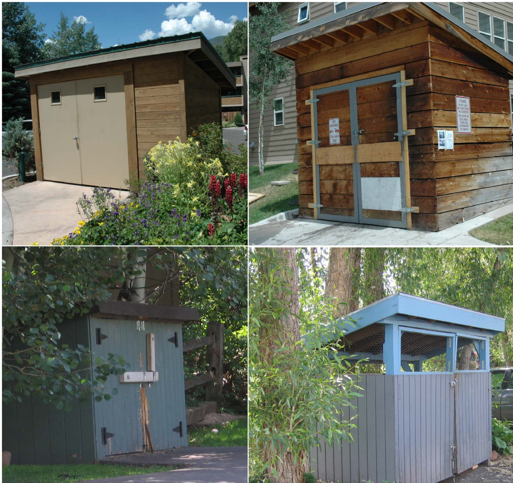
Fig. A4. Enclosure—Bear-resistant garbage containers secured by closed external doors of the structure, which at times allowed for non-bear proof containers to be stored securely inside. There were a variety of enclosure types: fully closed with building-grade constructed walls and metal doors which proved difficult for bears break into (top-left), fully closed with wooden side walls and/or front door, which bears were able to break into (top-right and bottom-left), and semi-open enclosures which were poor in preventing bears from obtaining garbage (bottom-right). There were also many enclosure latching methods including round door knobs (top-left), slide bar (top-right), and drop bar (bottom-left). We note that the most robust enclosure design was a well-constructed room with metal front door and round doorknobs like the enclosure in the top-left panel.
